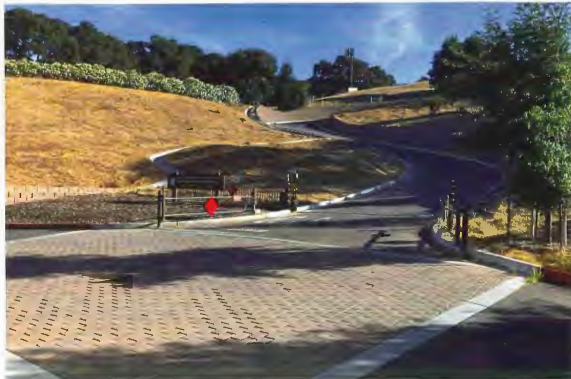
Elworthy Staging Area Las Trampas, Danville Parking 0.12 mi. in. Elevated and obscure
